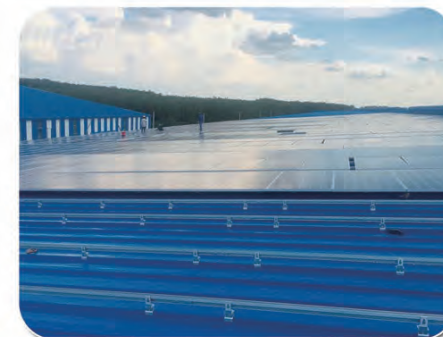
4 MW SFS-PR-01 Tin Roof Clamp Racking (Vietnam)
